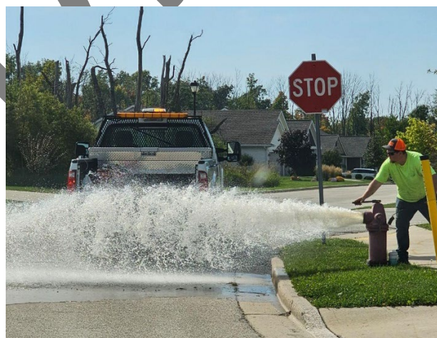
Employee performing regular hydrant flushing
