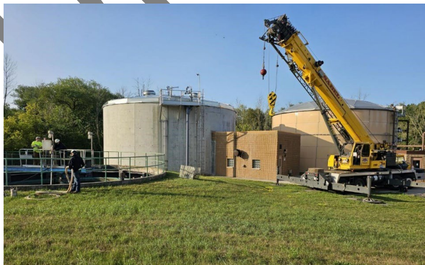
Village Wastewater Treatment Plant
