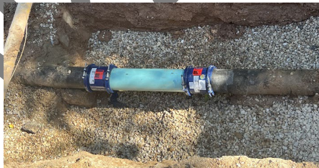
Exposed water main repair
