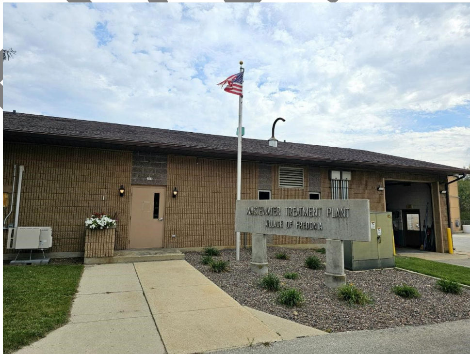
Village Wastewater Treatment Plant
