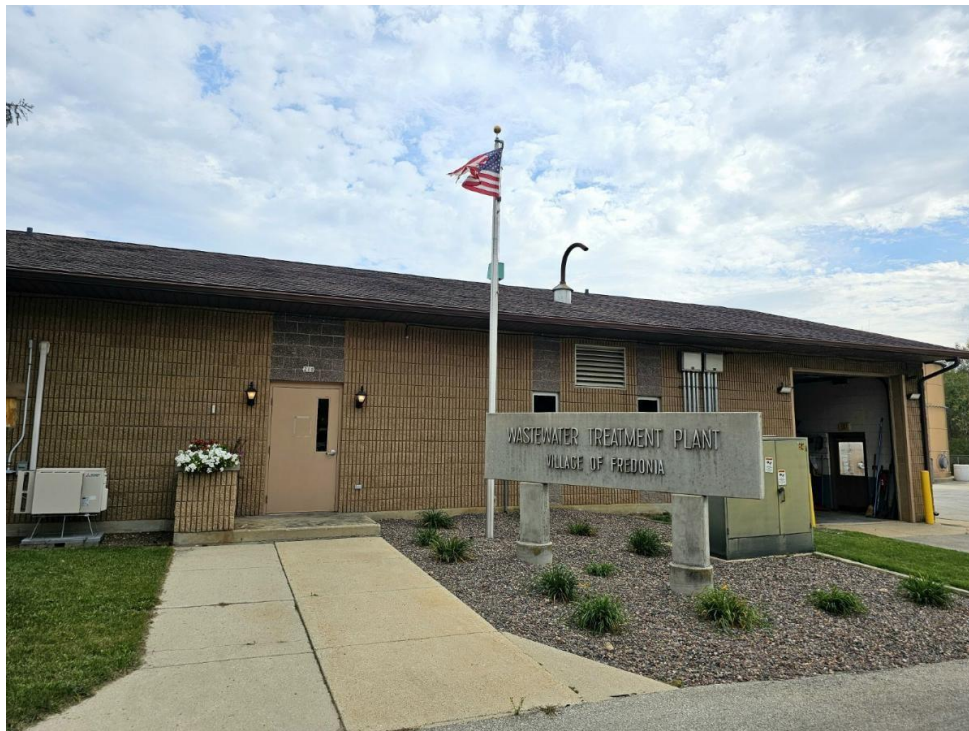
Village Wastewater Treatment Plant
