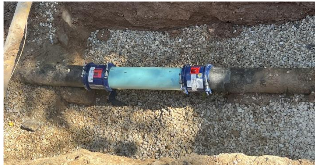
Exposed water main repair
