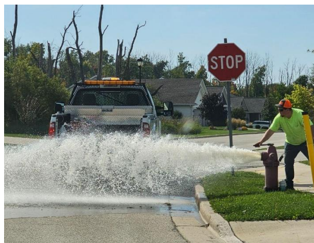
Employee performing regular hydrant flushing
