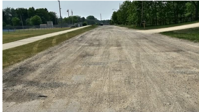
Newly paved surfaces such as Wilson St (shown left) received a PASER rating of “10”, where as crumbling roads such as Wisconsin St (shown right) are a “1”.
